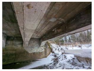
West beam exhibiting cracking, delamination and spalling along length.
