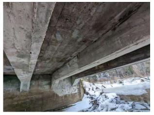
Deck soffit, isolated concrete patchwork.
