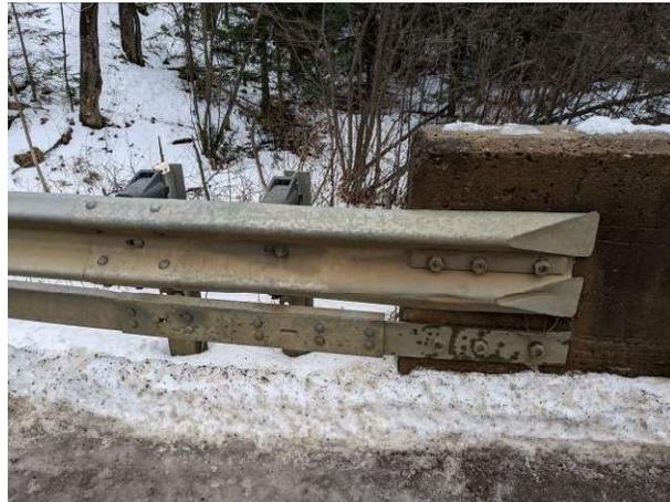
Coatings breakdown on anchor bolts.
