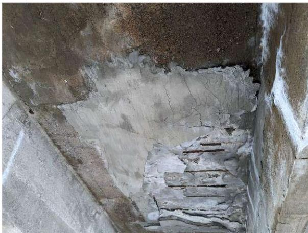
Deck soffit, interior. Concrete patchwork delaminated and spalled.
