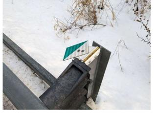
Reflector signage damaged.
