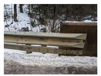
Coatings breakdown on anchor bolts.
