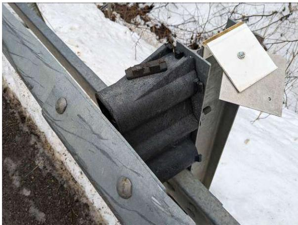
Offset block damaged and loose.
