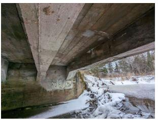
Deck soffit, isolated concrete patchwork.
