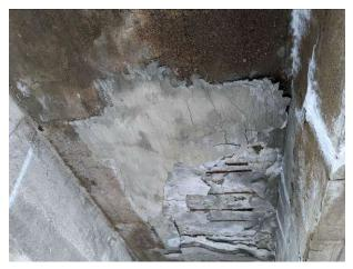
Deck soffit, interior. Concrete patchwork delaminated and spalled.
