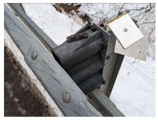
Offset block damaged and loose.
