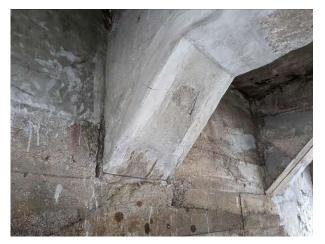
Beam end, south side. Cracking and delamination in concrete patchwork.
